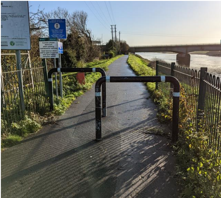
Figure 4-2: Example of Chicane Barrier (Barrier 3)
